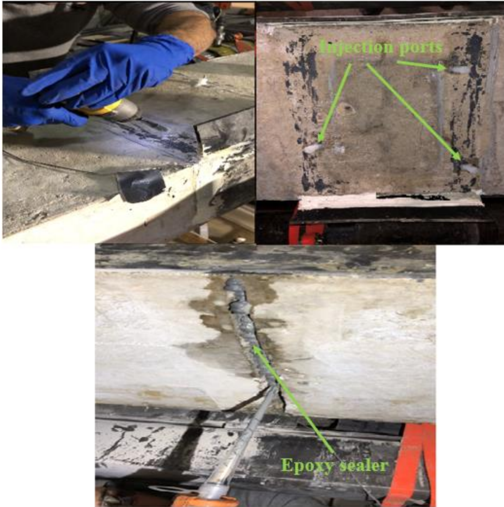
Figure 3-29: Installation of the injection ports on top of the holes and sealing the bottom surface of the NC panel at crack location
