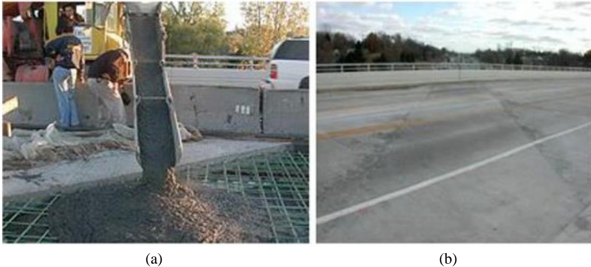
Figure 2-13: ECC link slab of Grove Street Bridge, Michigan, USA a) ECC casting b) Finished surface (Qian et al., 2009)
