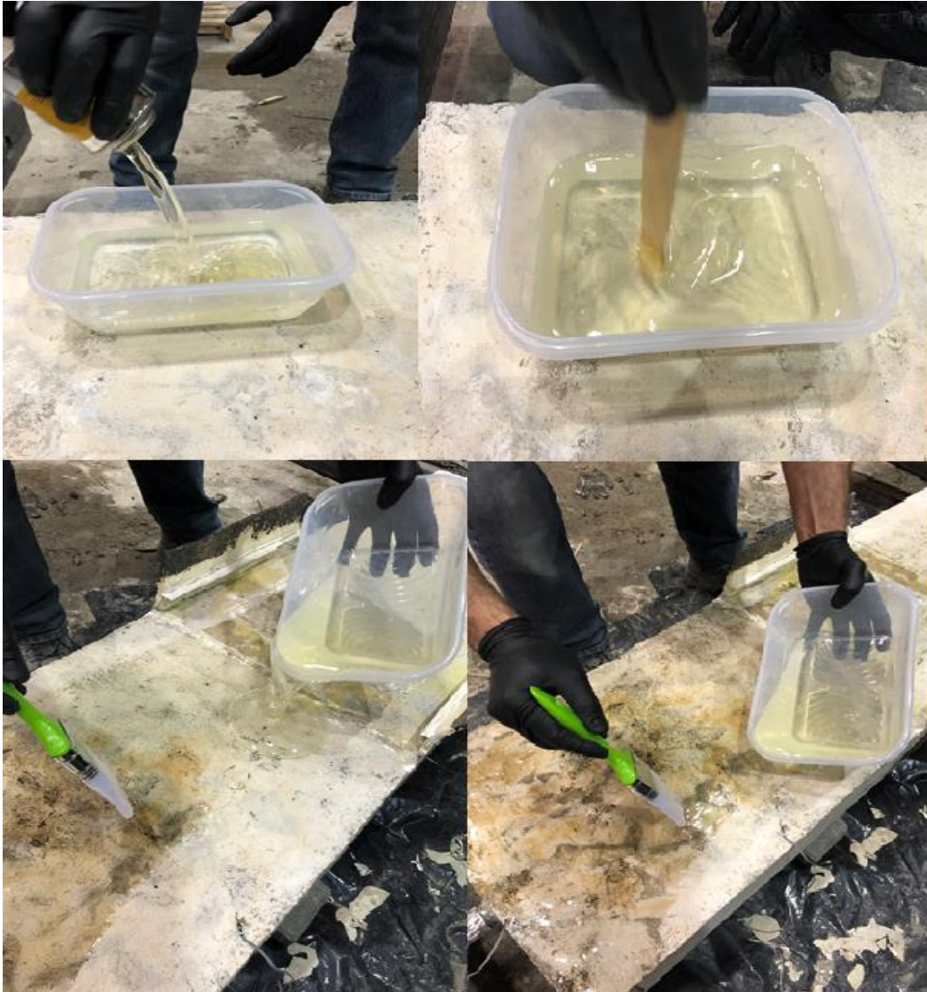
Figure 3-33: Mixing the resin and hardener and applying the epoxy resin system on the top surface of the RC panel
