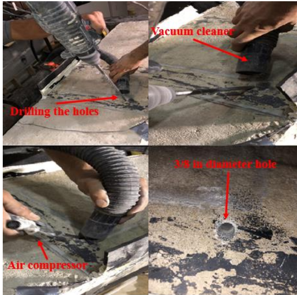
Figure 3-28: Procedure of drilling the NC panel and removing the dust using vacuum cleaner and air compressor
