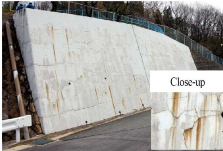
Figure 2-8: Deterioration due to Alkali-silica reaction (ASR) in a gravity retaining wall in Gifu, Japan (Rokugo et al., 2005; Yeganeh, 2013)
