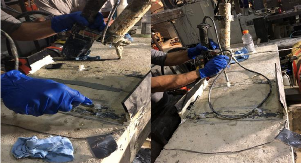
Figure 3-30: High-pressure epoxy injection
