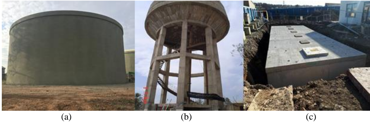
Figure 4-35: Classification of the tanks based on placement condition: a) Resting on the ground b) Elevated c) Underground
