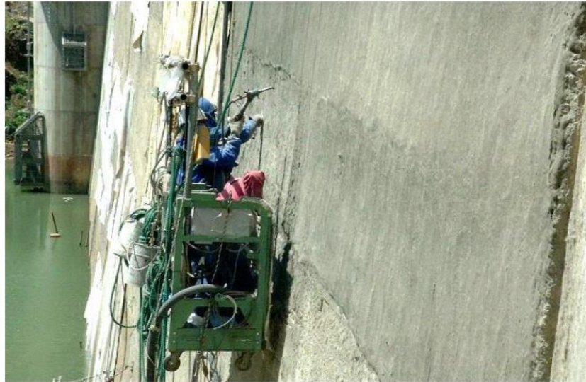
Figure 2-12: Water-proofing of Mitaka Dam in Hiroshima-Prefecture, Japan in 2003 by spraying ECC repair layer (Kojima et al., 2004)
