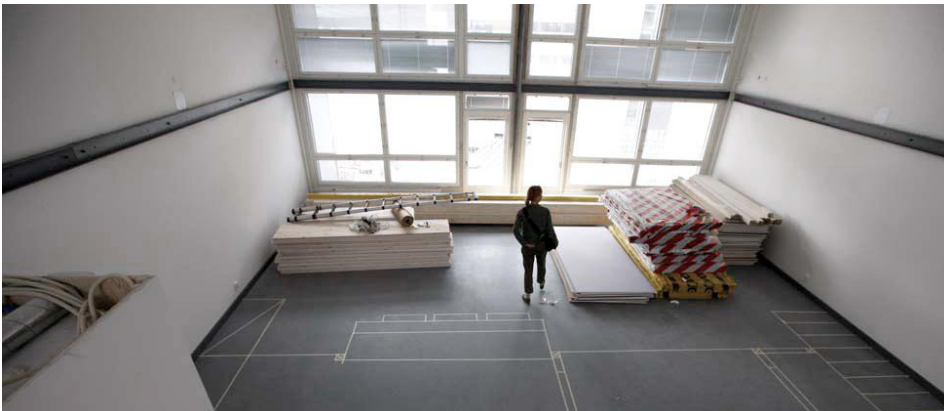
Figure No.6-6 Tila Housing Project by Talli Architecture, 2010, Helsinki, Example of Open Building project. Image showing in progress construction of Infill Level
