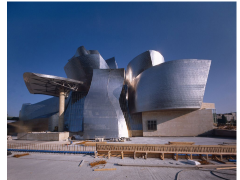
Figure No.1-3 Guggenheim Museum Bilbao by Frank Gehry, 1997, Bilbao, Spain. Using digital manufacturing techniques to fabricate the free form cladding
