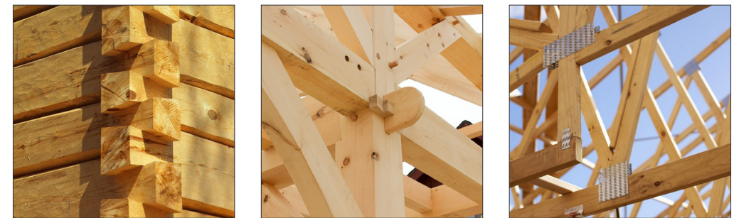
Images 23-25: Examples of cross-log, timber-frame, and stick-frame wood joints
