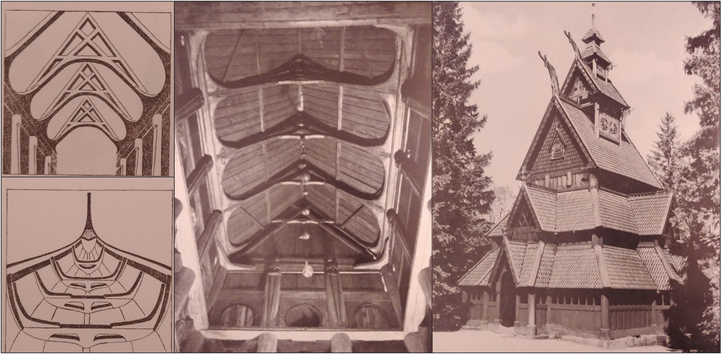
Image 5: Norwegian ship and roof frame comparison (left) Image 6: View of stave church roof truss from the interior (center) Image 7: Exterior stave church (right)
