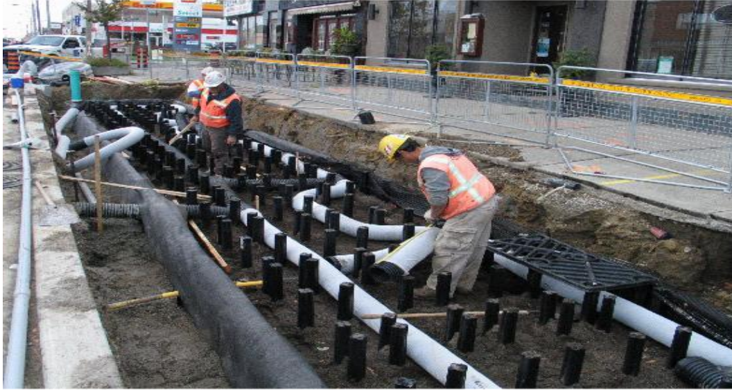
Figure 2-5 Installation of underground Bioretention System [2]
