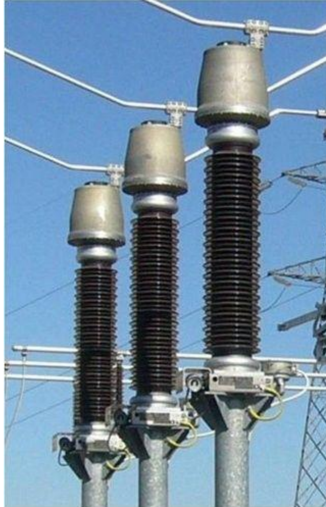
Figure 21: Voltage transformer in substation
