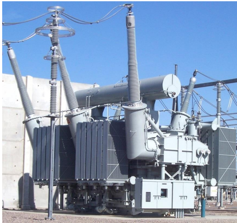
Figure 53: Power transformer
