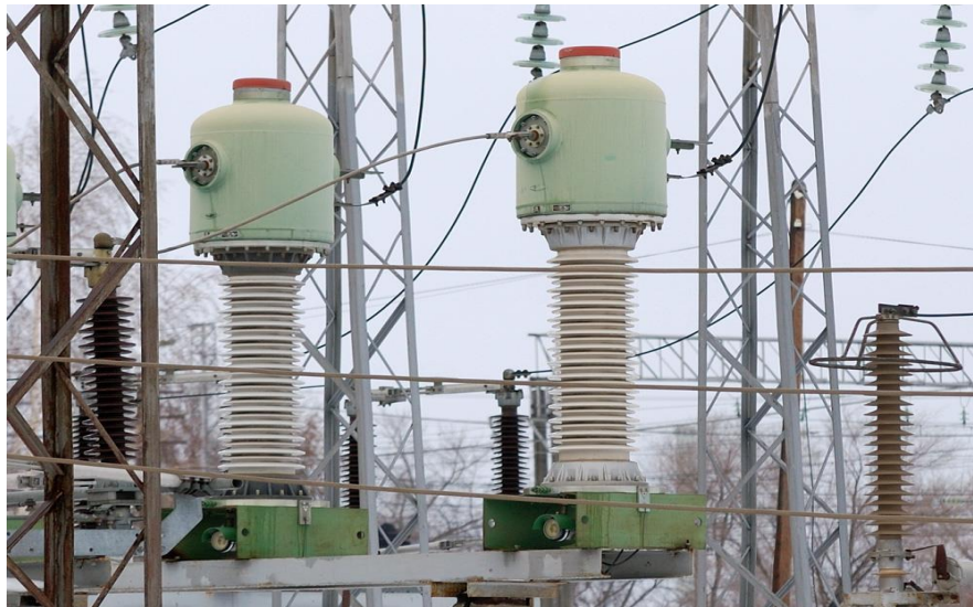
Figure 16: High Voltage Current transformer
