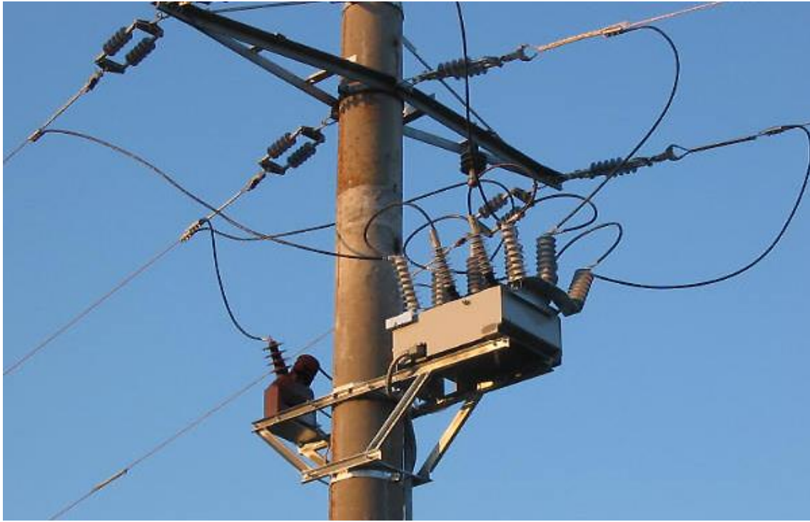
Figure 29: Automatic Circuit Reclosers
