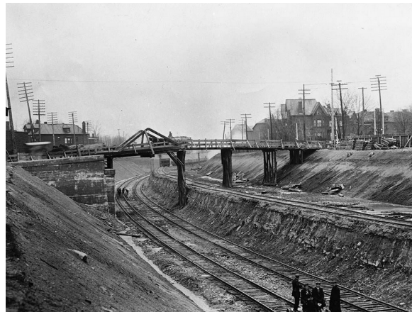
Figure 8 Temporary wooden bridge used during grade separation activities, Jameson Avenue (1911)
