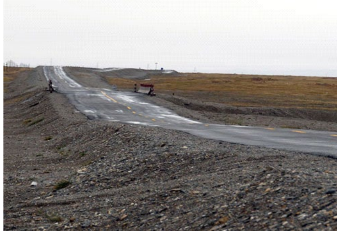
Figure 2: Uneven permafrost melting causing road damage, Tibet (National Snow and Ice Data Centre, 2013)
