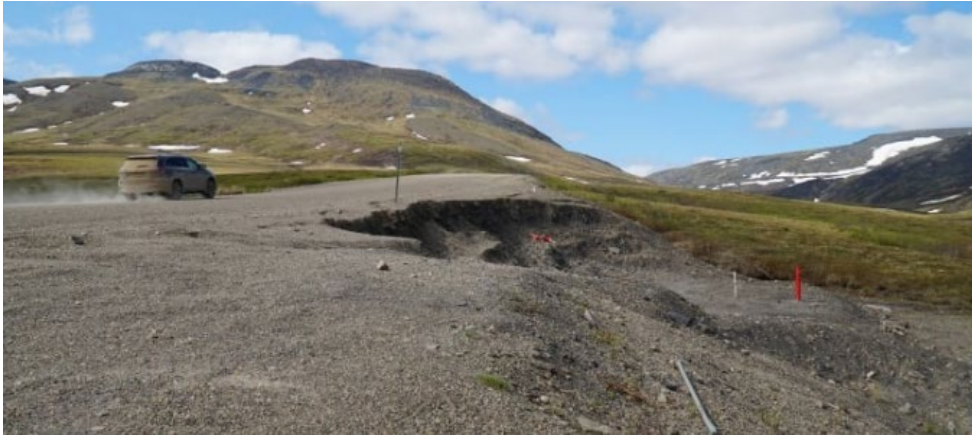
Figure 1: Landslide and erosion of road embankment along the Dempster Highway (Ormiston & Sheldon, 2019)
