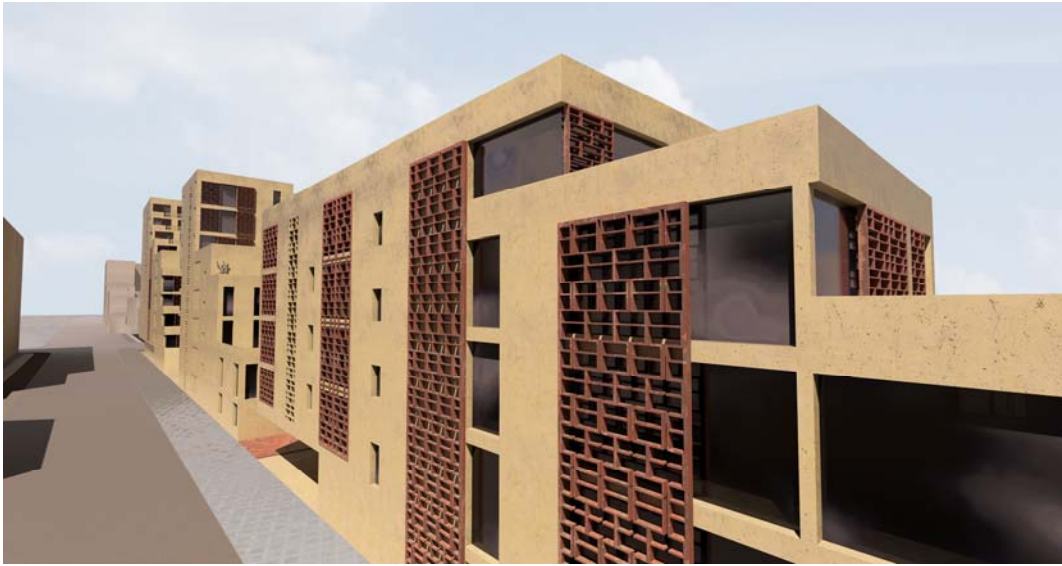
Figure 83: Proposed shadings for south side of the buildings. Source: Author
