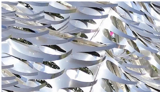
Figure 3-7 Thermobimetal panel for the Bloom pavilion
