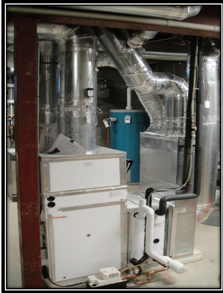
Figure E.4 – Air handling unit for the Archetype Sustainable House-B
