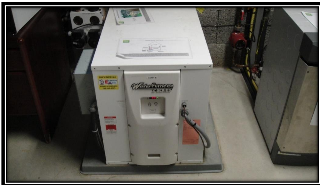
Figure E.5 – Ground source heat pump for the Archetype Sustainable House-B
