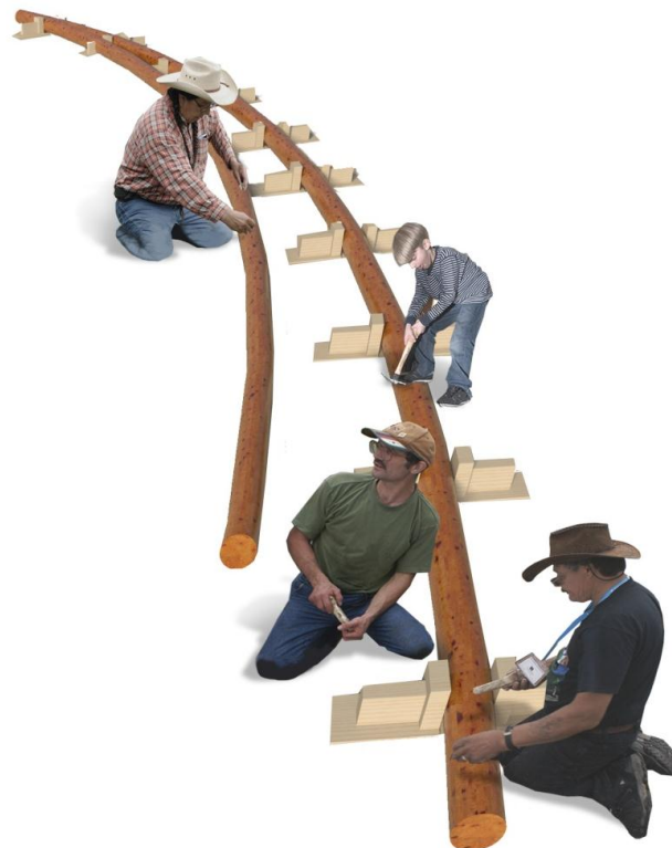
Figure 3.29 Constructing truss out of curved Spruce saplings using form-work
