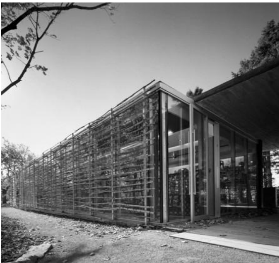
Figure 49: Deliberate fabrication with the use of lashed tree branches
