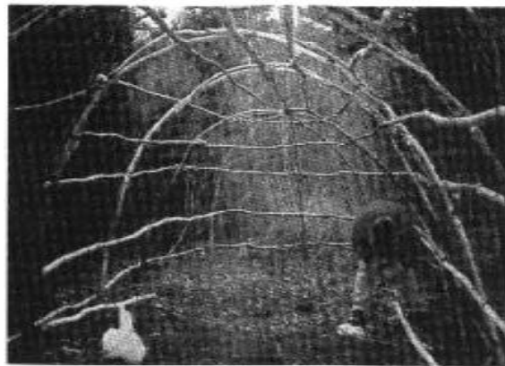
Figure 45: Traditional bent wood tensile framing (ceremonial structure)
