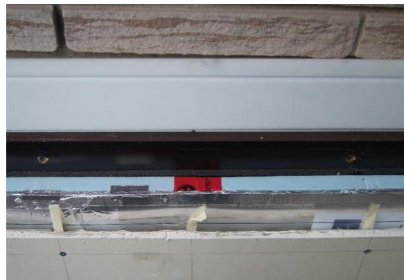
1) Ceiling structure of the composite PCM test cell
