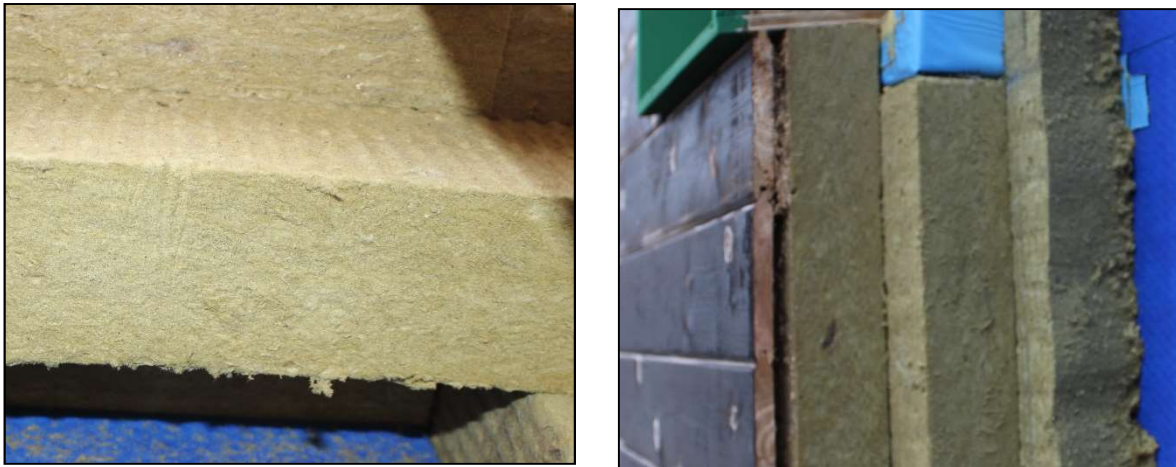
Figure 4-7 : Exterior Insulation Layer Interfaces
