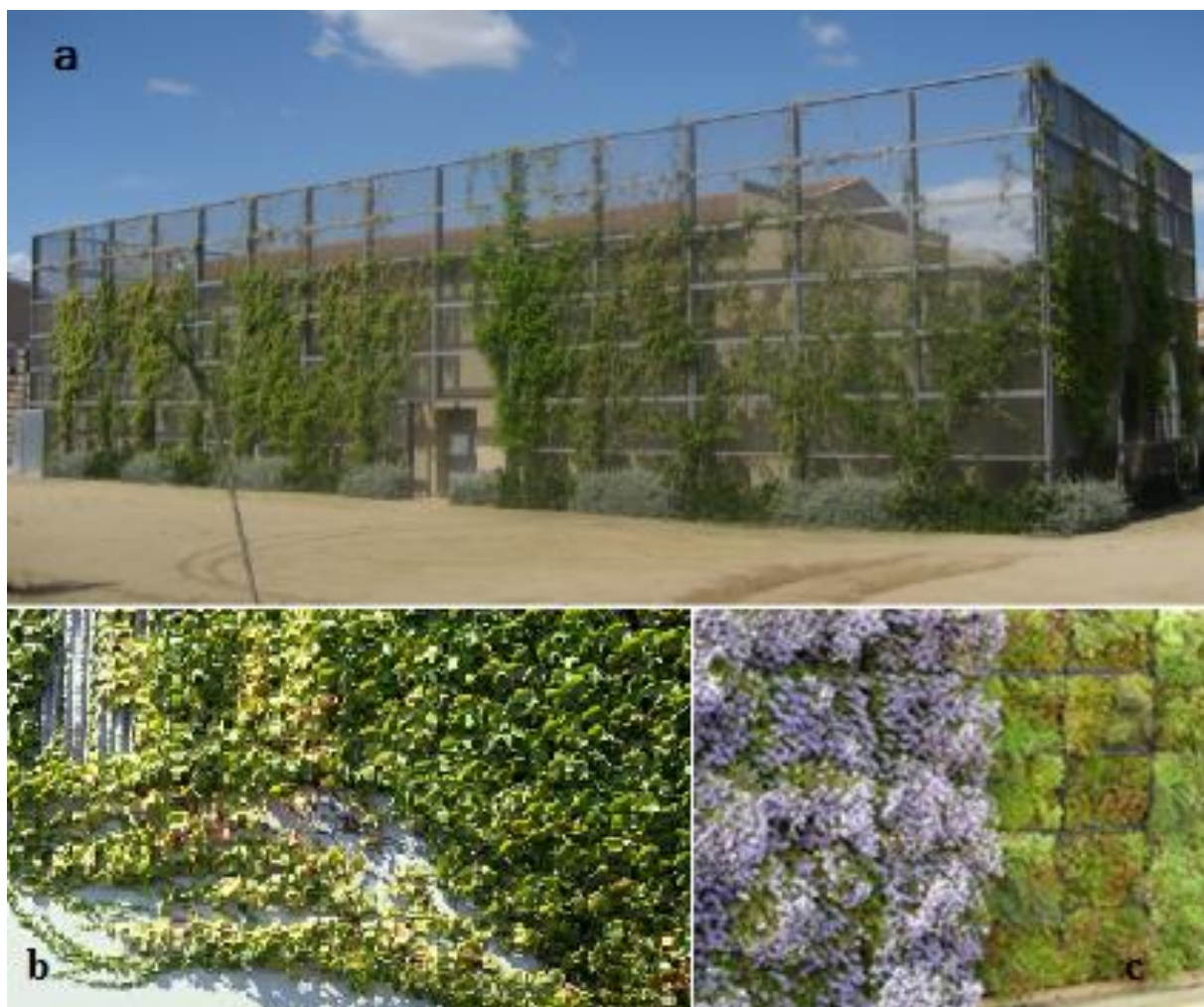
Figure 2.3: Categories of green walls: a) green façades (Pérez et al., 2011), b) traditional (PNW Plant Disease Management Handbook, 2013) and c) living walls (Perini et al., 2013).
