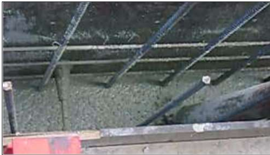
Fig. 2.1: Self-consolidating concrete construction (www.oboa.on.ca)
