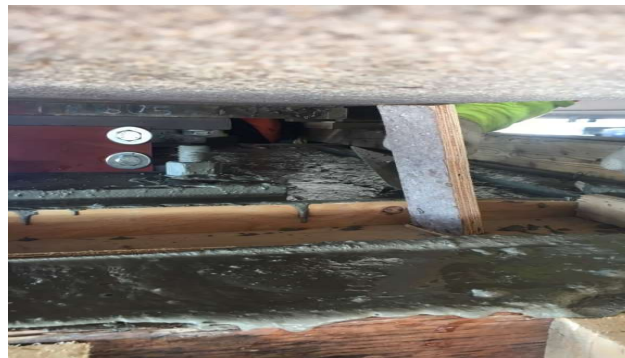
Fig. 2.2: SCC used as a bridge bearing pad on Highway 7/400, Vaughan, ON
