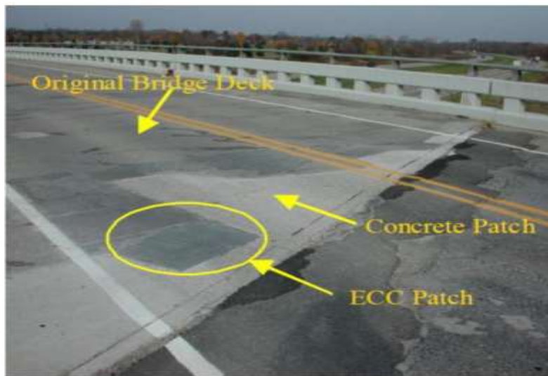
Fig. 2.7: ECC patch repair on Michigan bridge deck (Li et al., 2005)
