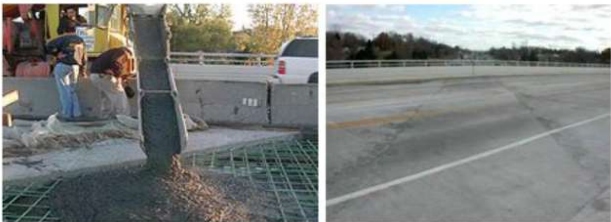
Fig. 2.8: ECC link-slab on Grove Street Bridge, Michigan (Qian et al., 2009)
