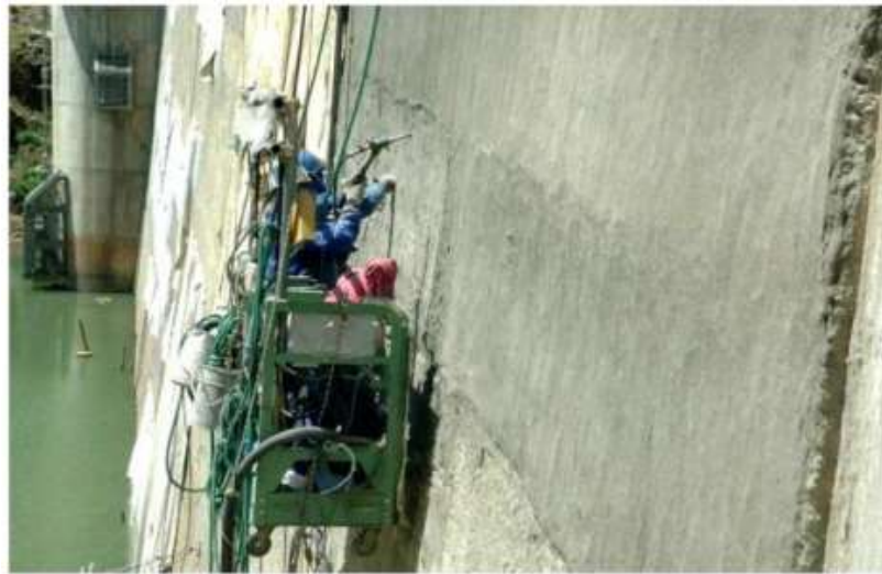
Fig. 2.5: Spray repair of the Mitaka dam with ECC for water-proofing (Sakata et al., 2004)
