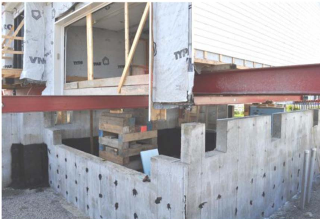
Figure 1 - 3: Replacement procedures for the foundations and walls [2]
