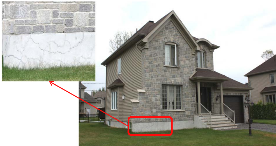
Figure 1 - 1: Cracking in concrete foundation [2].
