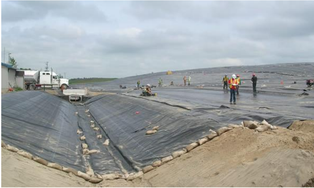
Figure 5.4. Interim Capping of the Trail Road Landfill (J.L. Richards & Associates, 2011)
