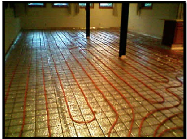
Figure 4.26: Hydronic flex tubes laid out on floor assembly and heat reflectors
