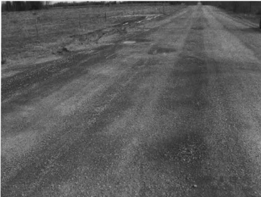
Figure 4.30: Road Surface without Shingles after six months
