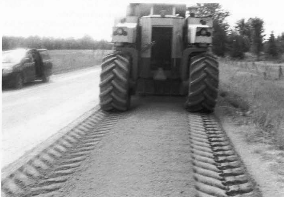
Figure 3.9: Pulverization of Existing Gravel Road
