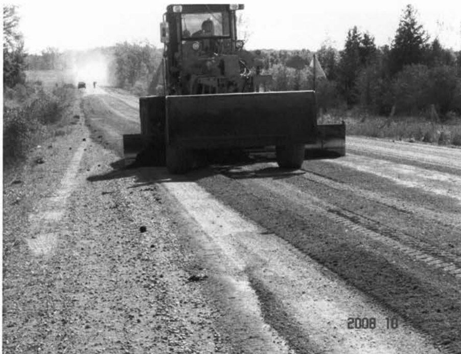
Figure 3.14: Mixing of Shingles and Gravel with Grader
