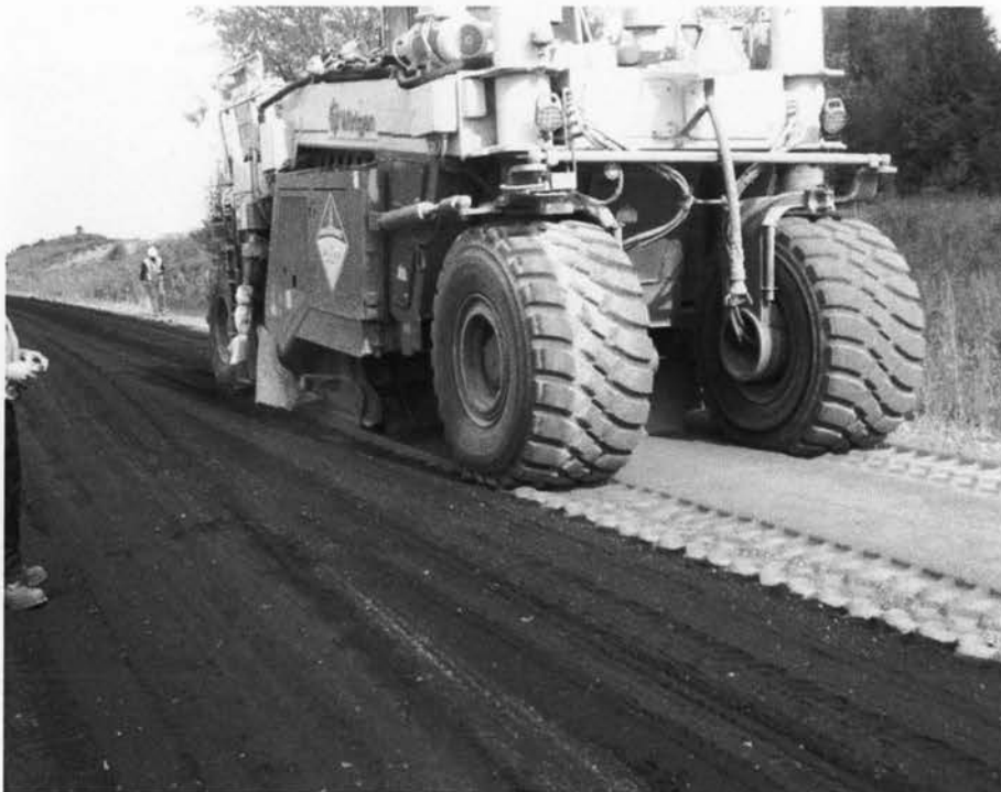
Figure 3.13: Mixing of Shingles and Gravel with Pulverization Machine
