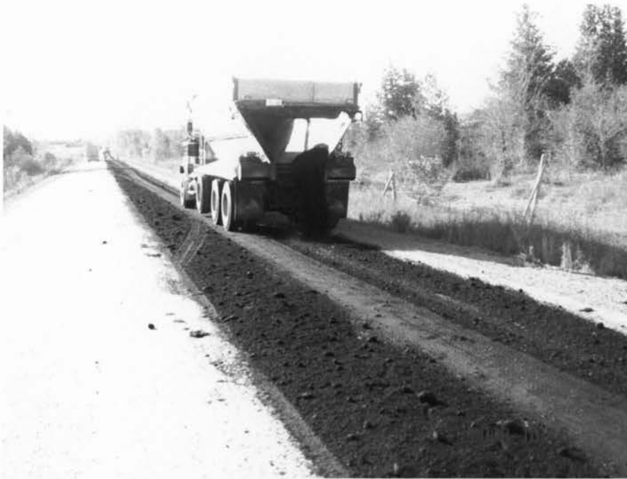
Figure 3.10: Placing Processed Shingles
