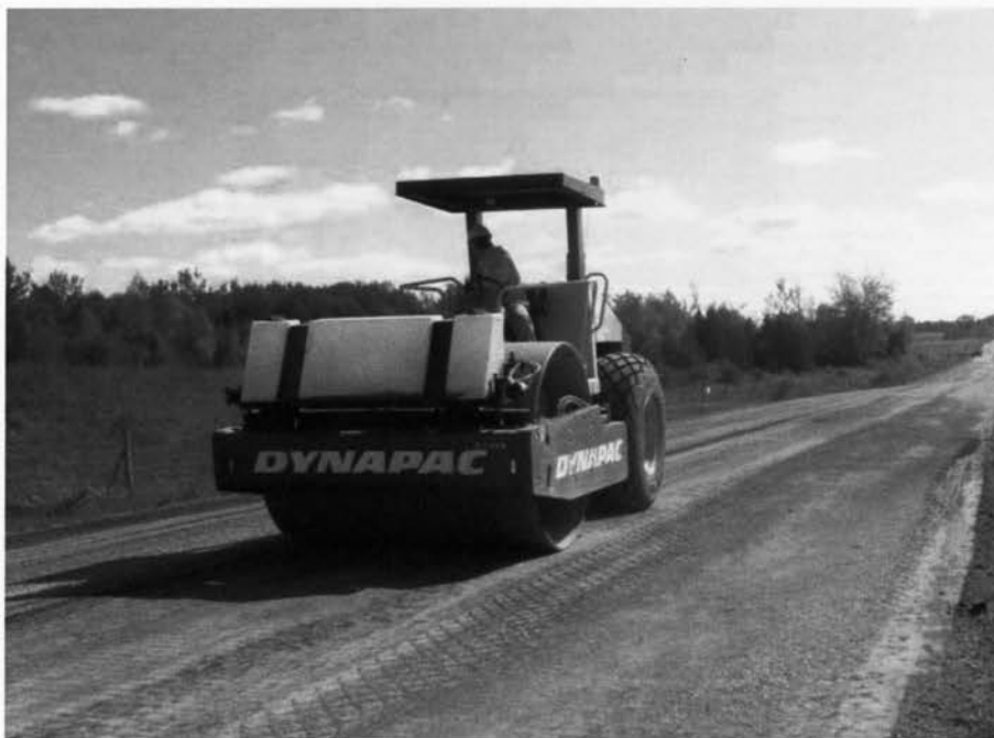
Figure 3.15: Compaction of Gravel
