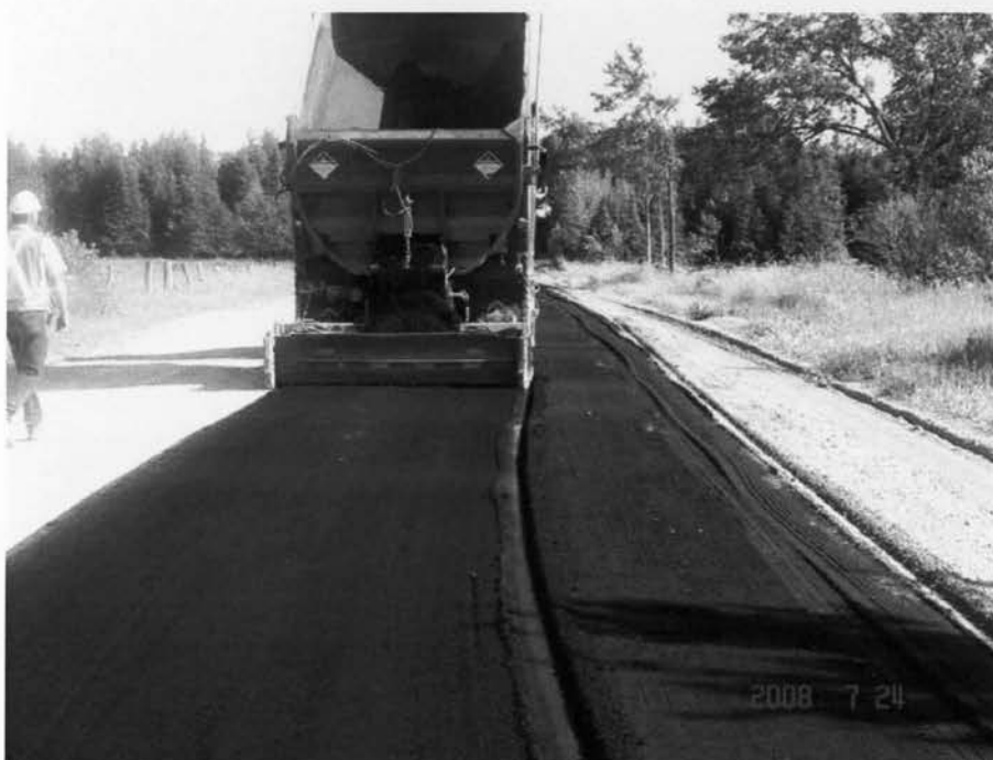
Figure 3.8: Spreading of Ground Shingles
