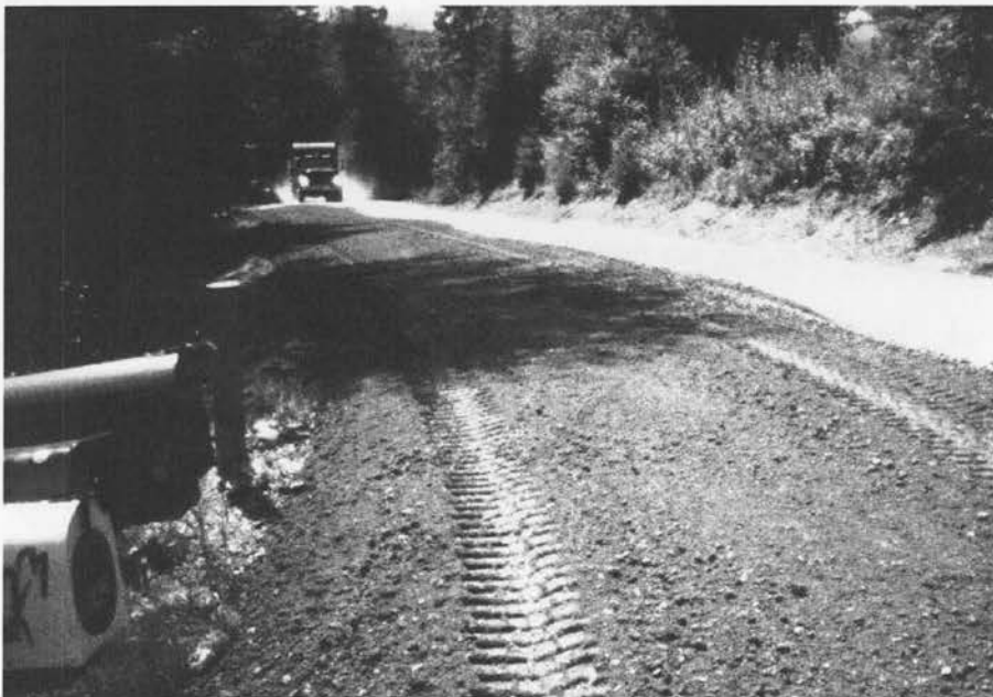
Figure 2.7: Shingles Mixed with Granular Material on TH17, Hinesburg (Source: Surwilo, 2003)
