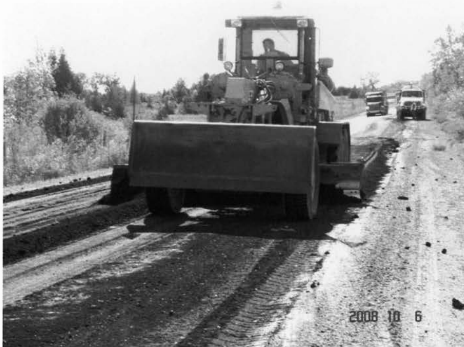
Figure 3.11: Spreading of Processed Shingles by Grader
