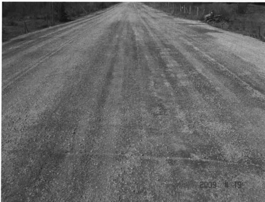
Figure 4.31: Road Surface with 12% Shingles after six months
