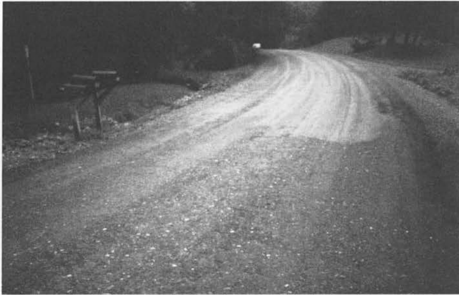
Figure 2.8: Shingles Mixed with Granular Material, TH17, Hinesburg (Source: Surwilo, 2003)
