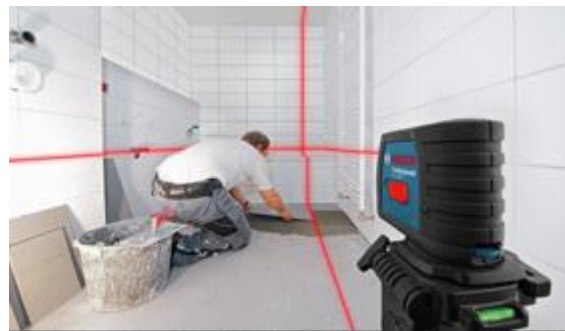
Figure 3-7. Laser line for perfect alignment.
