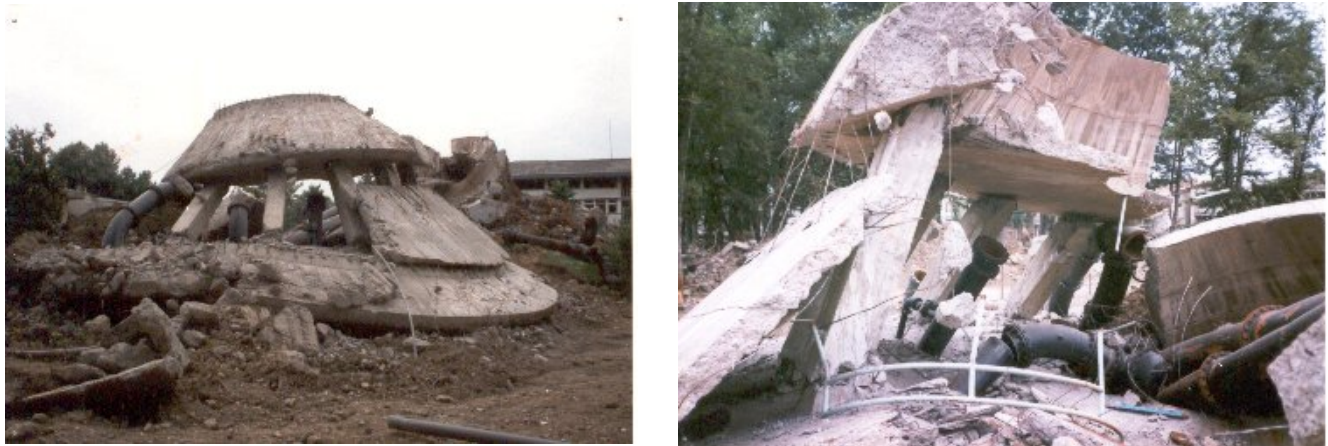
Figure 2.1 Debris and remaining of the collapsed 1500 m 3 water tower in Rasht during Manjil-Roudbar earthquake (Building and Housing Research Center, Iran 2006)
