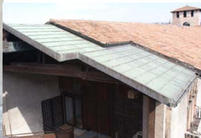
Fig. 1.7 Peeling Roof
