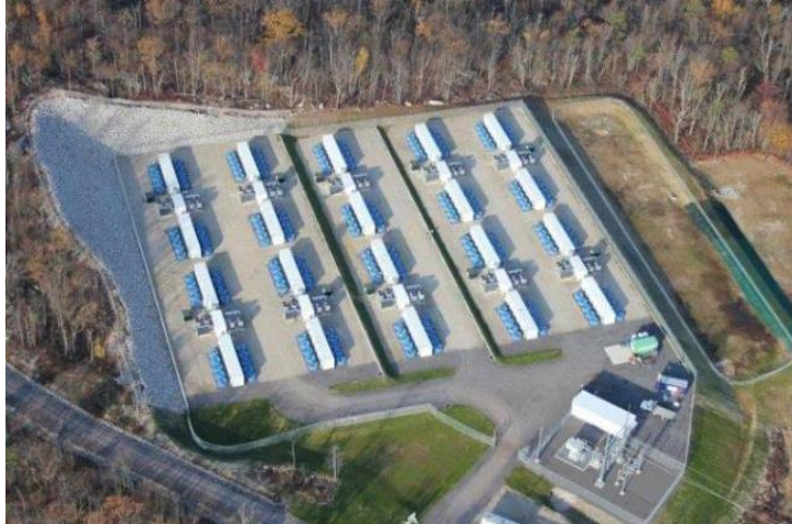
Figure 2.11: 20 MW Beacon Flywheel Power Plant, Stephentown, NY. Image taken from [Akhil, 2013].
