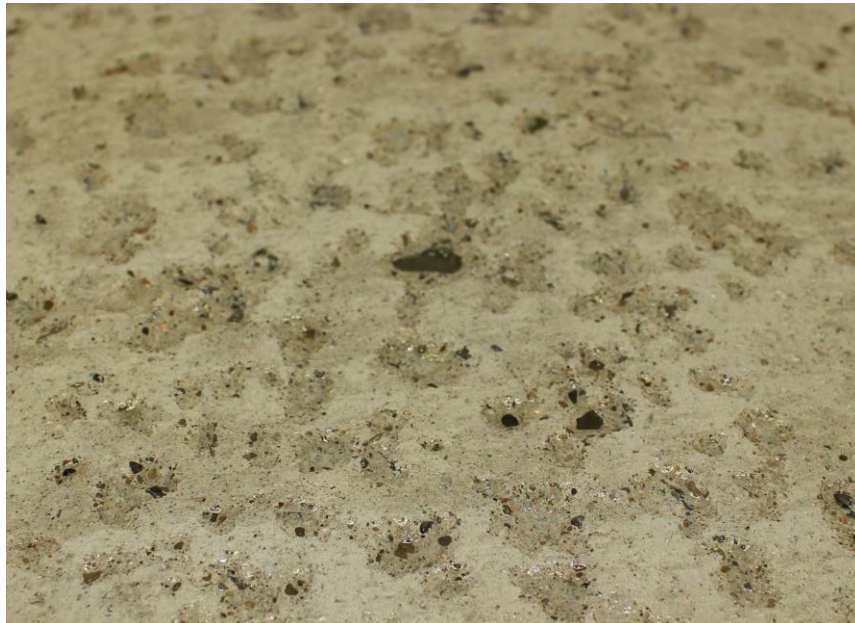
Figure 2.1-1: Salt scaling damage on surface of concrete.
