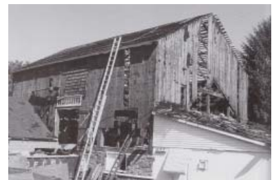
fig. 5.4.16 the barn in its original location Old surface coverings are revealed during dismantling.
