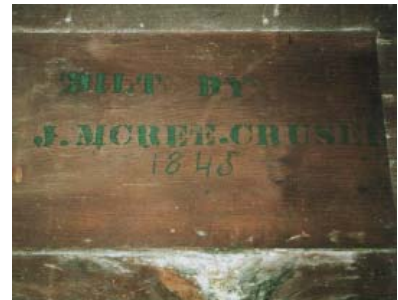
fig. 5.4.15 mr. mccree cruser Mr. McCree Cruser's name stenciled on a board used as a dutchman.
