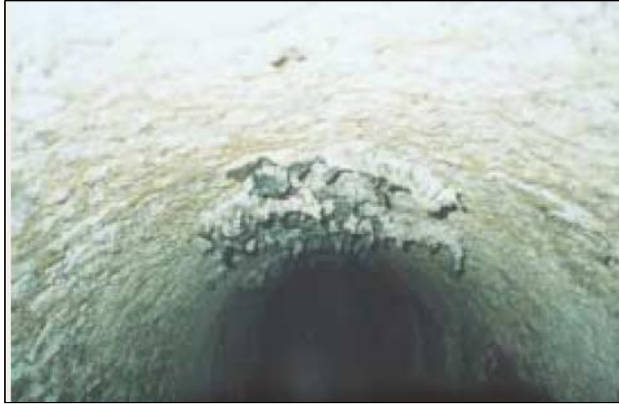
Figure 2.10 Hydrogen sulfide corrosion on the crown of a concrete pipe and the remains of the coal tar epoxy coating on the crown (Gebler 2003).
