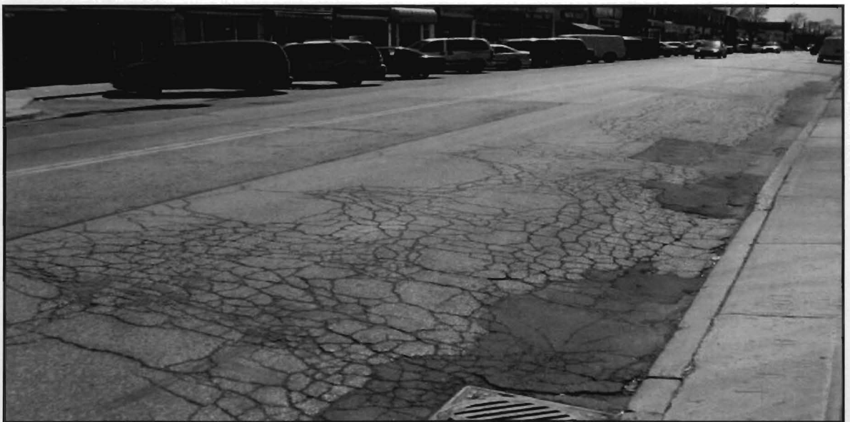
Figure 48: Pot holes and cracks at O' Connor & Donlands
