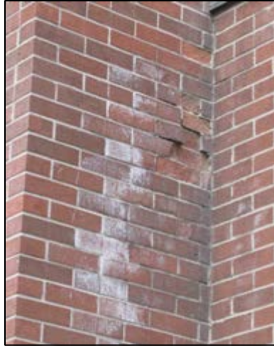
Figure 3 – Photograph of frost damaged brick masonry and efflorescence
