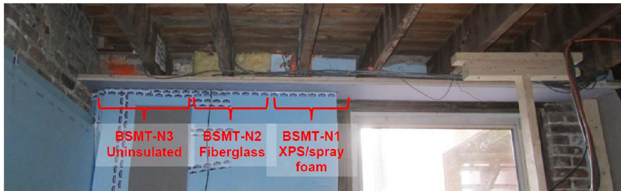
Figure 6: Comparison of Insulation Strategies for Heritage Masonry Buildings (Ueno, Straaten, & Schumacher, 2013)
