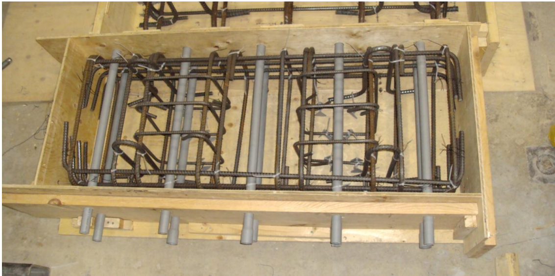
Fig. 4.19 Formwork and reinforcement cage, a) panel A, b) panel B, c) panel C, d) RC distributing beam
