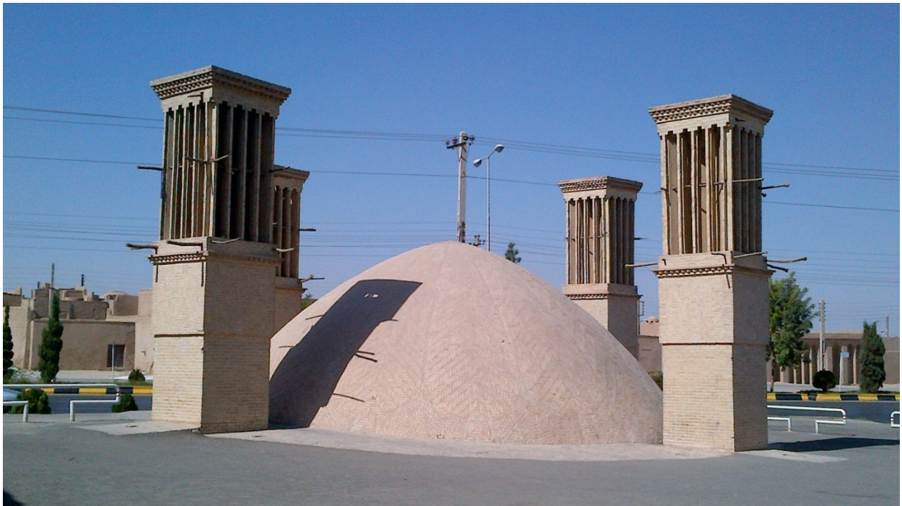
Char-Badgir Water Cistern – Yazd, depicting an ab-anbar surrounded by four cooling bad-gir
