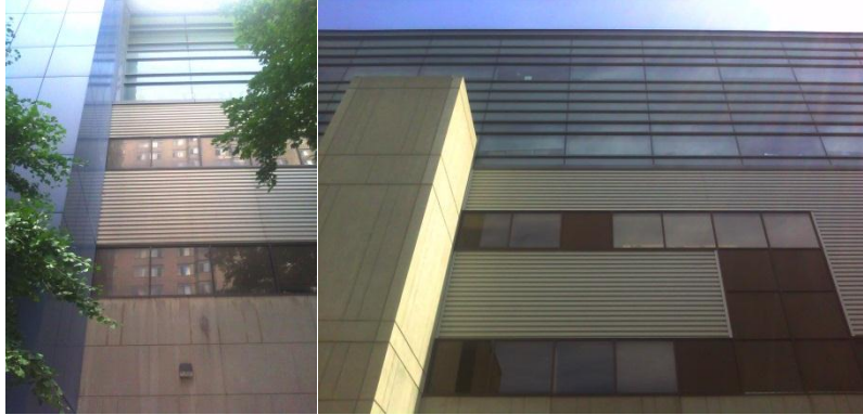
Figure 8: Mix of Cladding from various renovations to Eric Palin Hall/SHE
