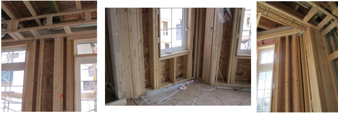
Figure 4.10: Door`s and window`s structural elements in the THs
