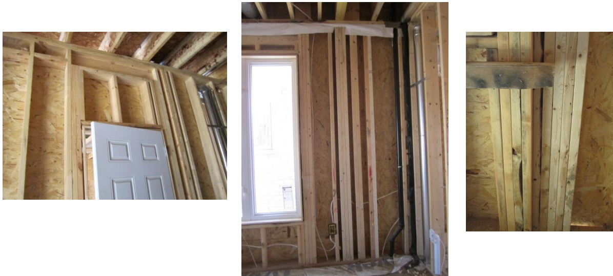
Figure 4.12: framing elements in some SDHs
