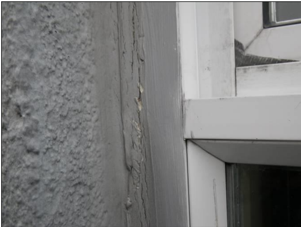
Figure 5 – Sealant deterioration around window frame (RDH, 2010)
