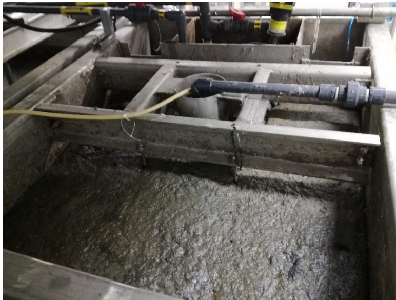
Figure 29: Rising sludge on the primary clarifier on Day 4 (Stage #6).
