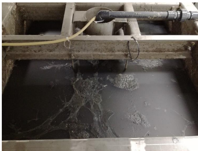
Figure 74: Film on the clarifier's surface after \text{NaHCO}_3 dosage.
