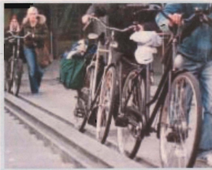
Figure 4.1.5.3. “Innovation in Mobility Management”, Here cycling to work is made easier by the wedges alongside the staircase. The wedges are there to support the bicycle as one moves up the staircase. This only but one example of the articulation of infrastructure in Amsterdam to support the expansion of cycling. (Ministry of Transport, Public Works and Water Management, 2009)
