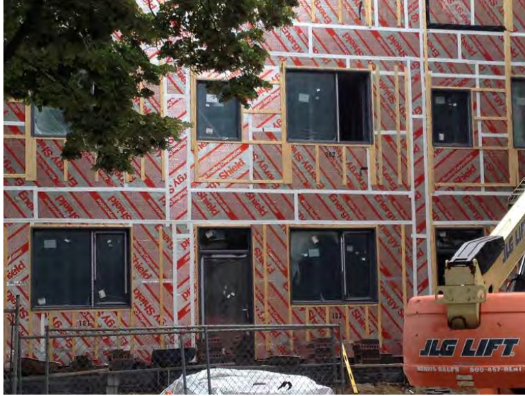
Figure 2-34 View of the seams sealed between the modules [McDonald, 2012]
