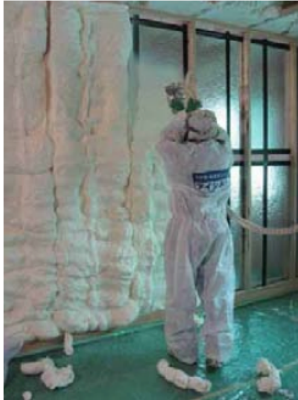
Figure 2-36 View of the spray foam over top of the VIPs [Parekh & Mattock, 2012]
