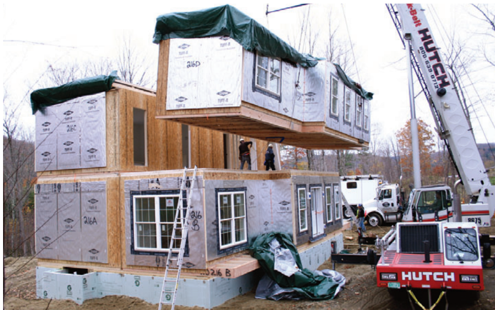
Figure 2-17 Modules installed on site for modular example #2 [Biebel, 2011]
