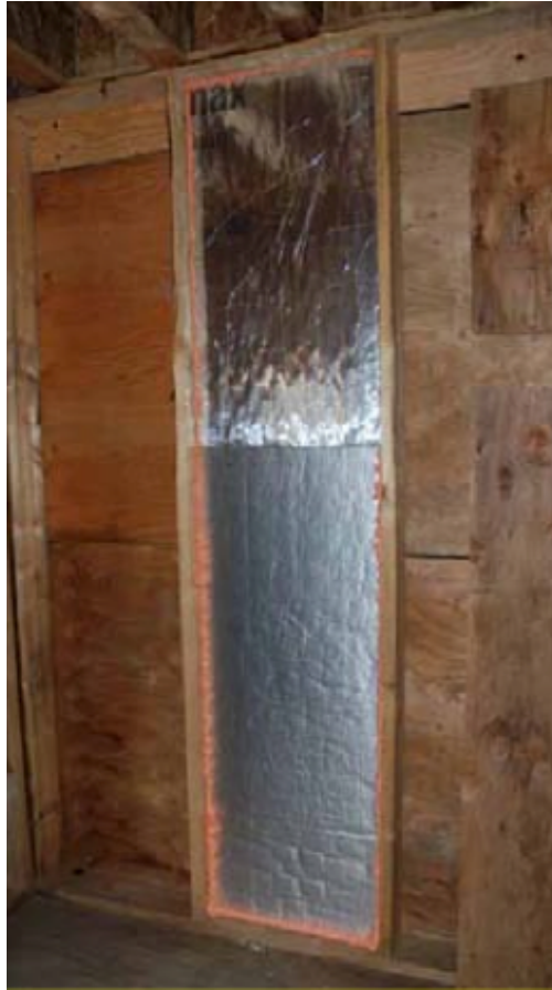
Figure 2-38 View of VIP located within the framed cavity [Parekh & Mattock, 2012]
