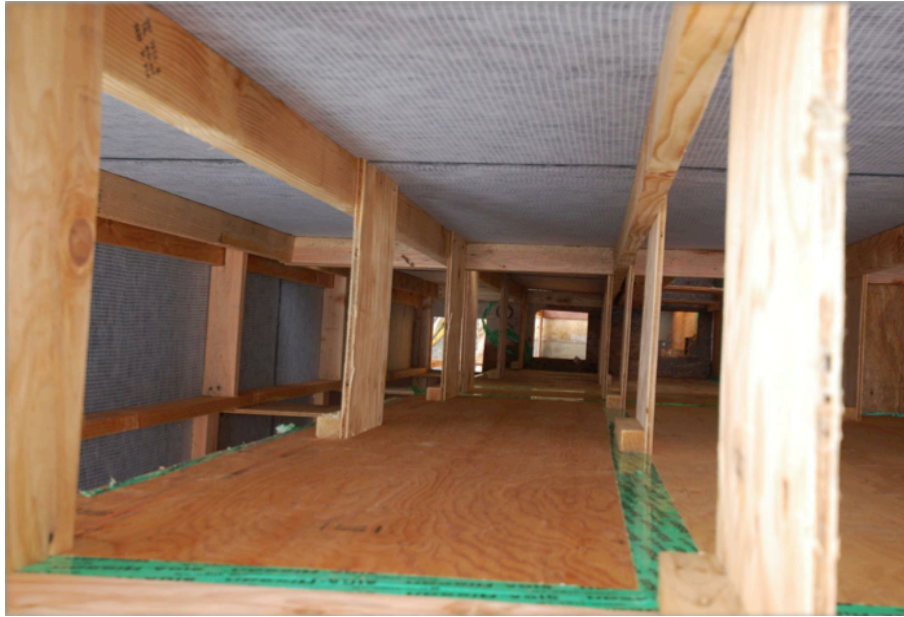
Figure 2-31 View from the top of a larson truss assembly [Clupp, 2012]
