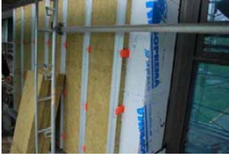
Figure 2-37 View of exterior applied VIP system [Parekh & Mattock, 2012]
