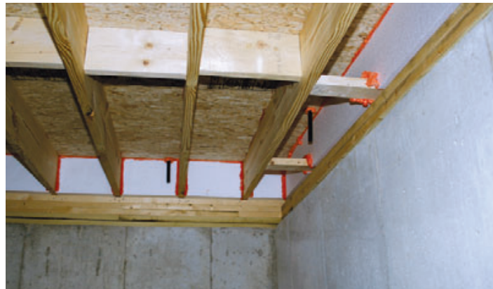
Figure 2-20 View of rim joist [Biebel, 2012]
