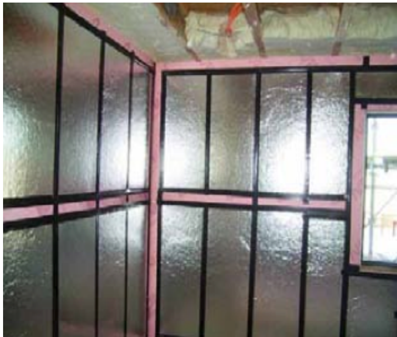
Figure 2-35 View of VIPs on interior side studs [Parekh & Mattock, 2012]
