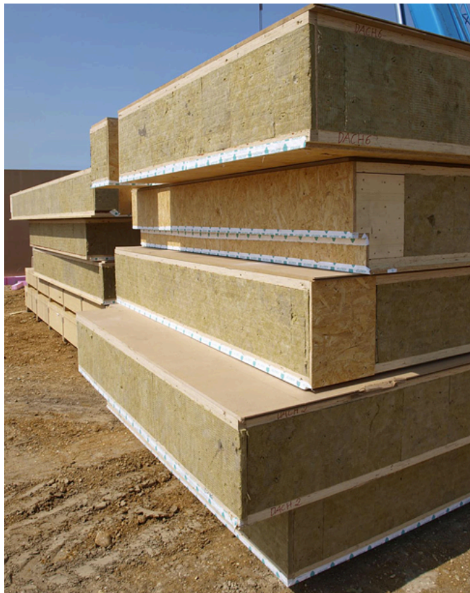
Figure 2-3 – Example of closed panelized envelope components [Brute Force, 2013]
