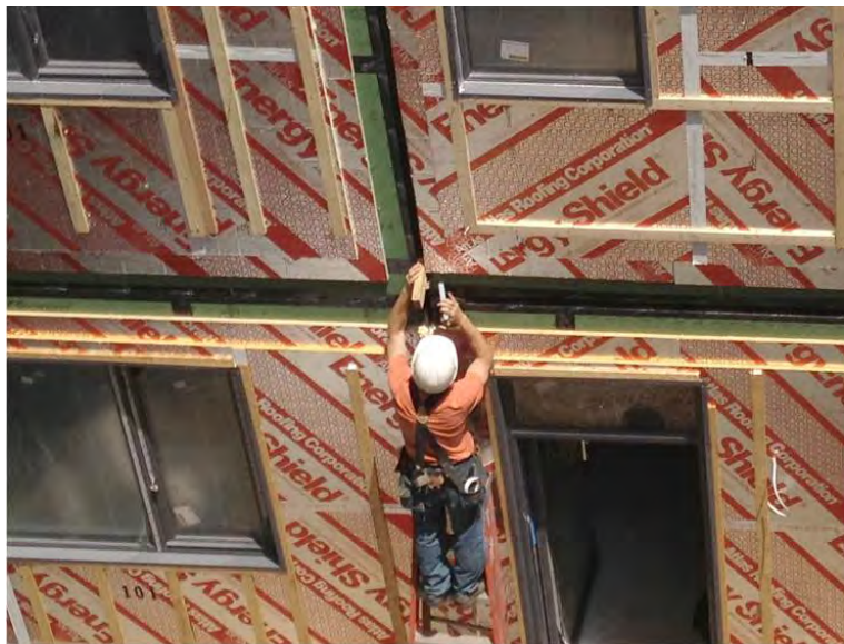
Figure 2-32 View of exterior applied polyisocyanurate assembly [McDonald, 2012]
