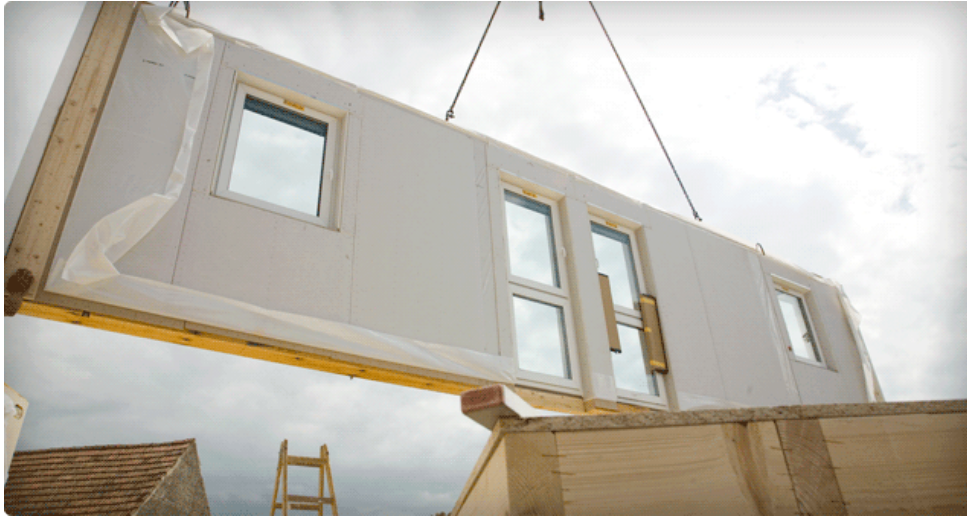
Figure 2-4 – Closed panelized system [Brute Force, 2013]
