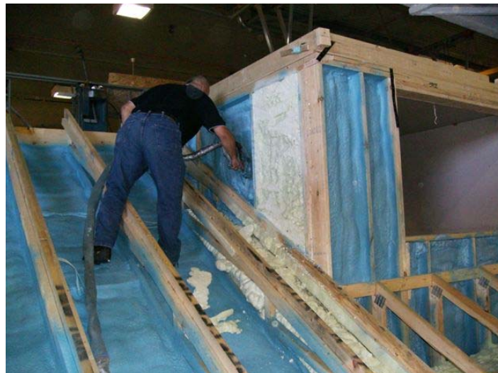
Figure 2-29 View of spray foam insulation in modular example #3 [Canadian Mortgage & Housing Corporation, 2011]
