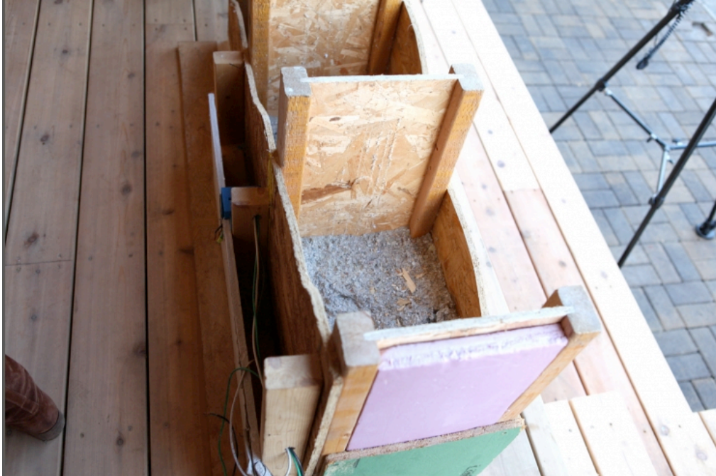
Figure 2-30 – Example of a vertical I-beam assembly [Klingenberg, 2012]
