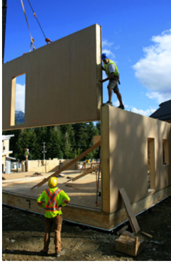
Figure 2-2 – Closed panelized system [BC Passive House, 2012]
