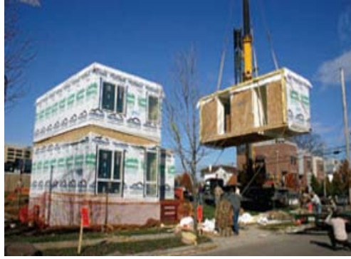
Figure 2-15 Module with WRB left open [NAHB, 2013]
