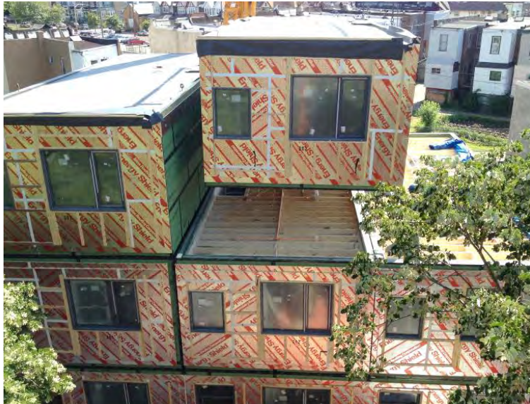
Figure 2-32 View of exterior applied polyisocyanurate assembly [McDonald, 2012]
