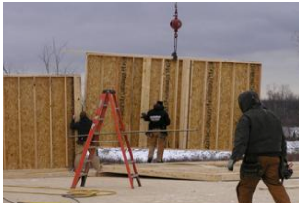
Figure 2-1 – Example of open panelized envelope system [Barden Homes, 2013]
