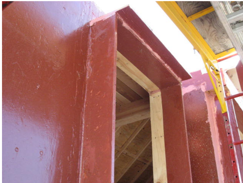
Figure 4-6 Liquid applied flashing around window buck [Prosoco, 2013]
