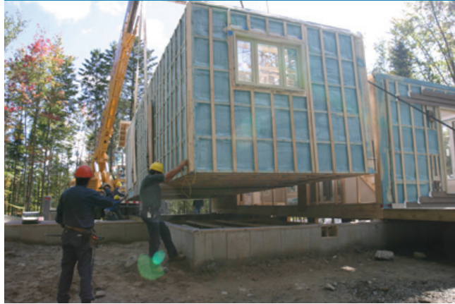
Figure 2-23 Module being installed for EcoTerra house [Canadian Mortgage & Housing Corporation, 2011]
