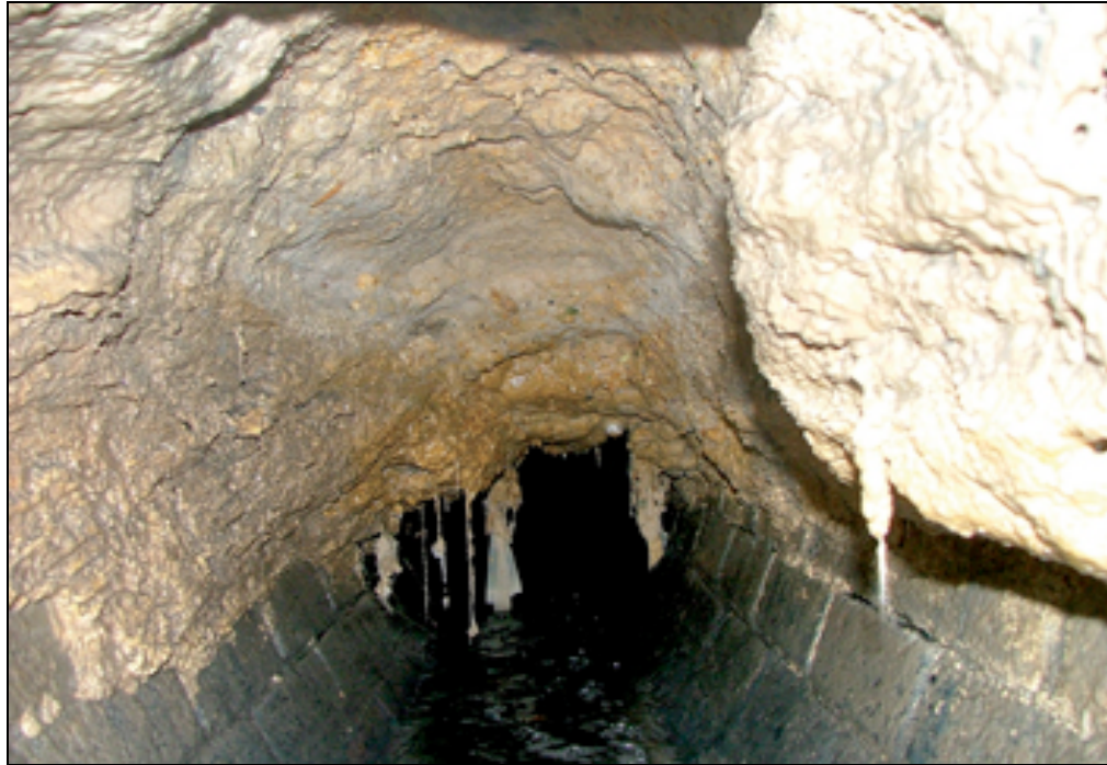
Figure 2.3 “Oily wastewater build-up” in sewer system
