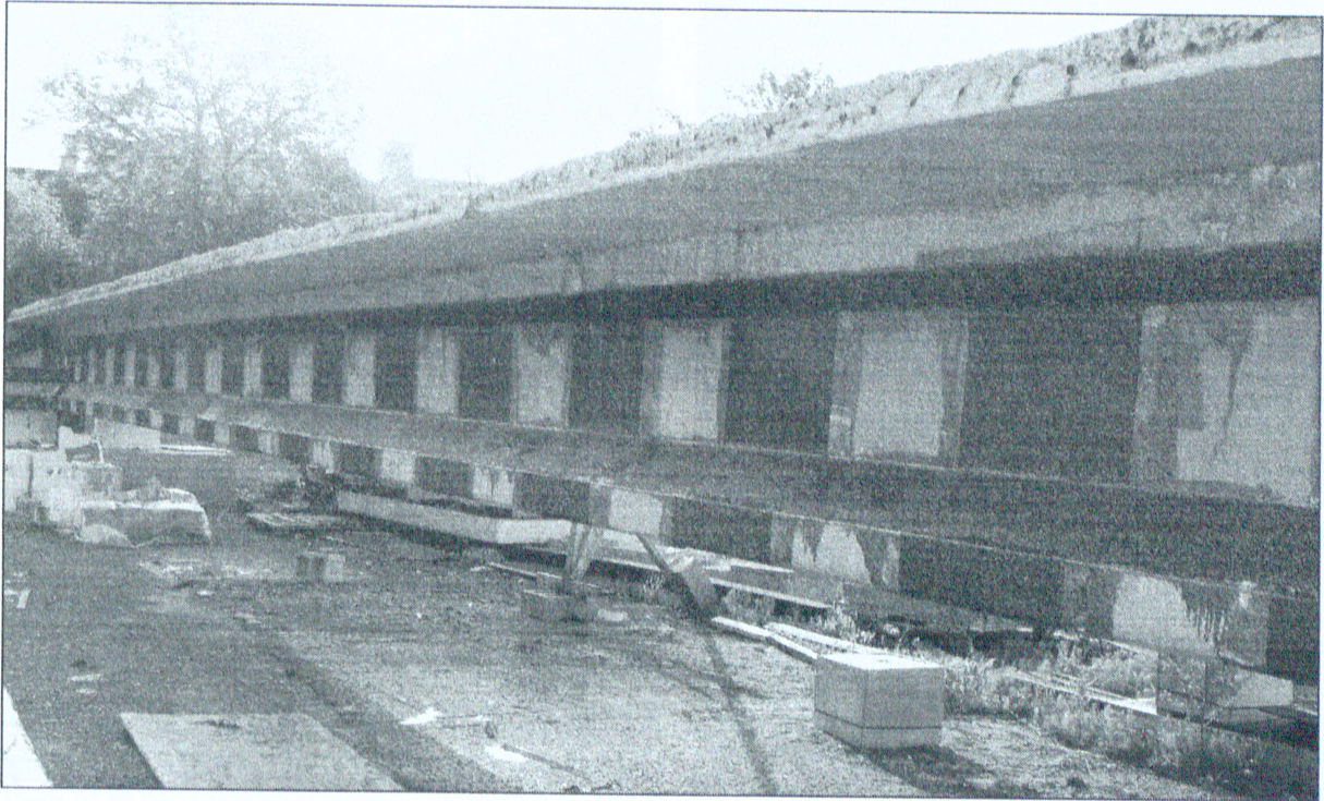
Figure 3.44 – Completion of one full layer of the CFRP system for entire girder length
