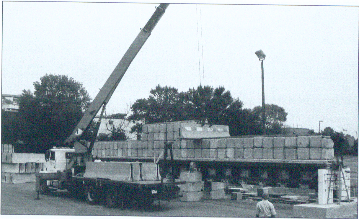
Figure 3.75 – Placement of first Jersey barrier
