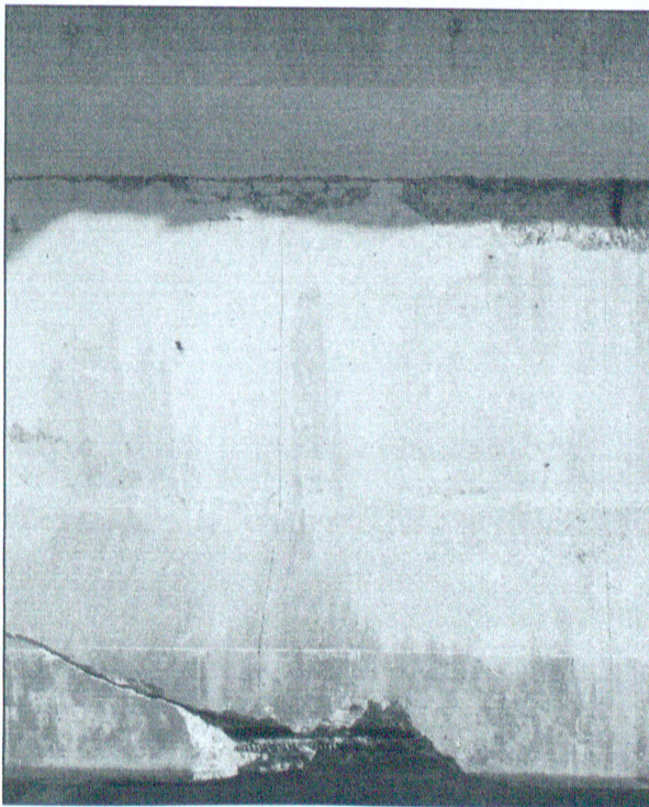
Figure 3.25 – Comparison of pre and post grouting for the south face
