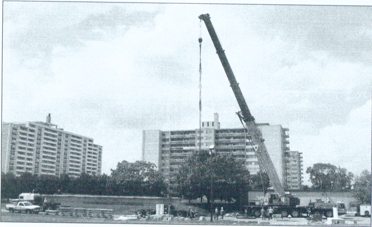
Figure 3.16 – Arrival of AASHTO Type III prestressed concrete girder
