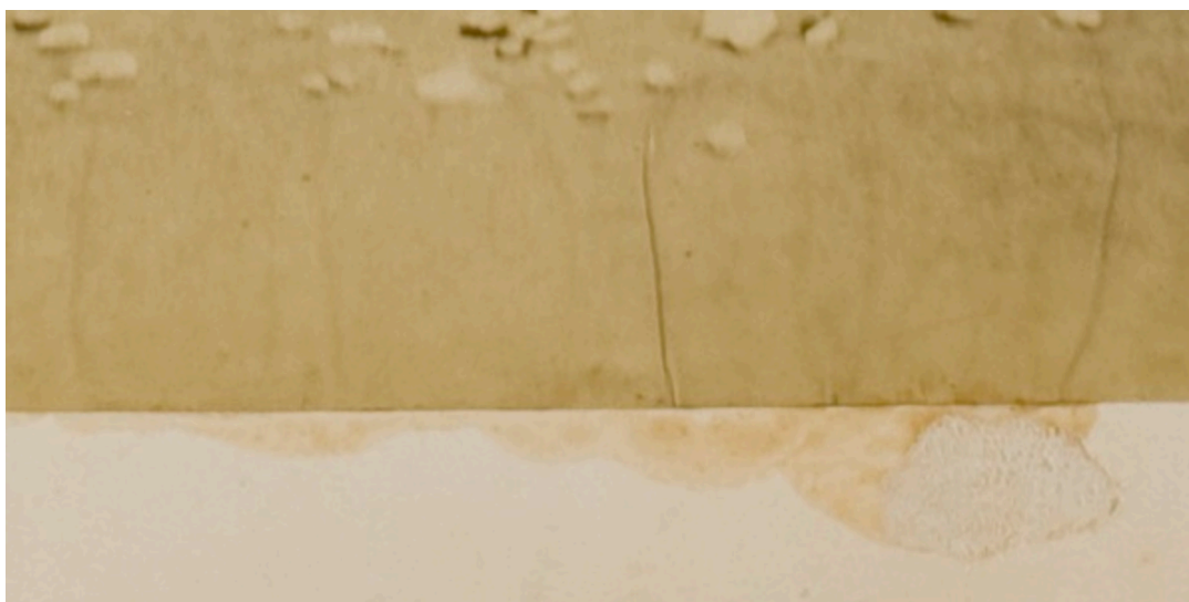
Figure 15: Poor adhesive technique
