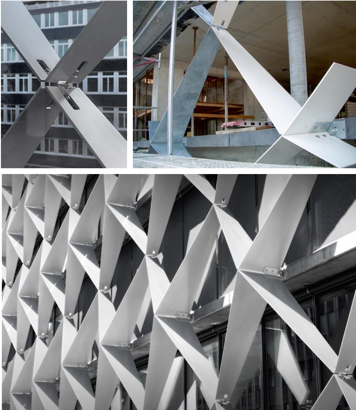
Figure 11: Diagrid Screen Connections, Dado House, Germany
