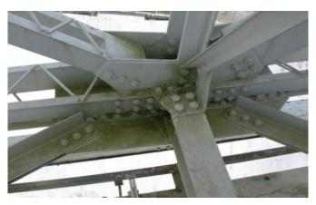
Figure 1-1: Bolted steel bridge connection made of structure steel (photo courtesy of KTA-Tator, Inc.)
