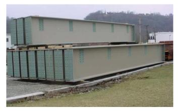
Figure 1-2: Steel main girder made from structure steel (photo courtesy of KTA-Tator, Inc.)
