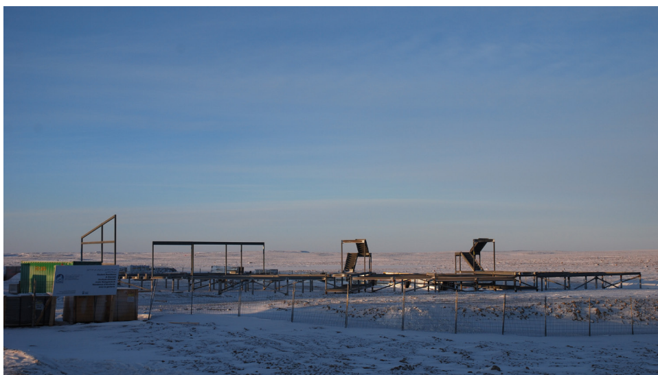
Figure 70: Steel Piles for the future Arctic College Building
