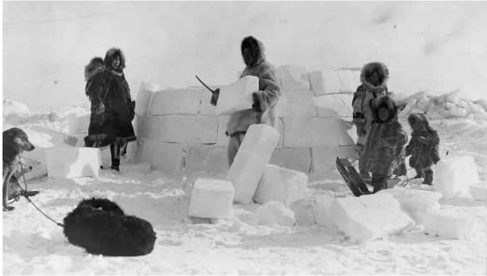
Figure 128: Igluit Construction
