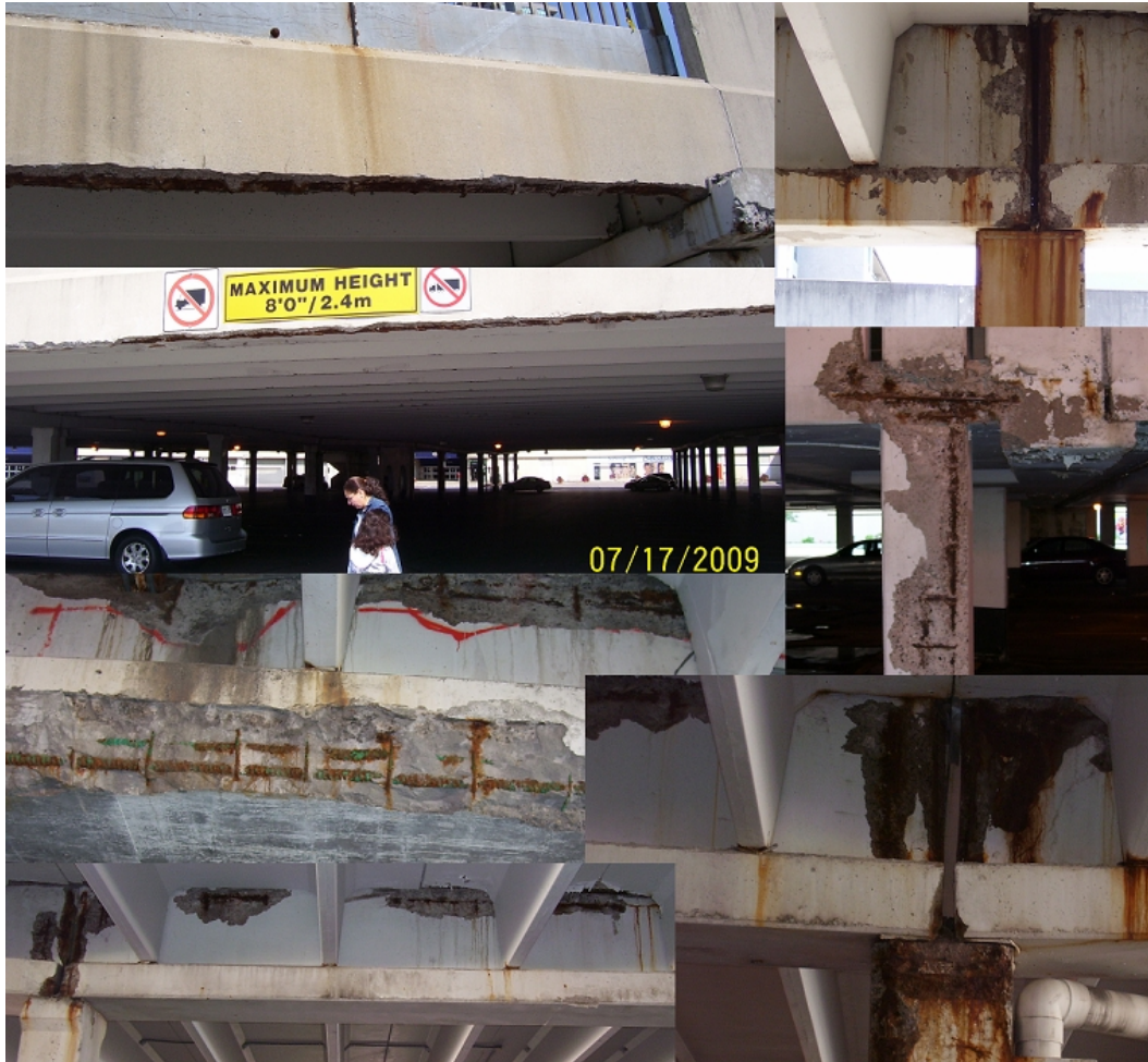
Figure (1-1): Corrosion damage in concrete beams and columns.
