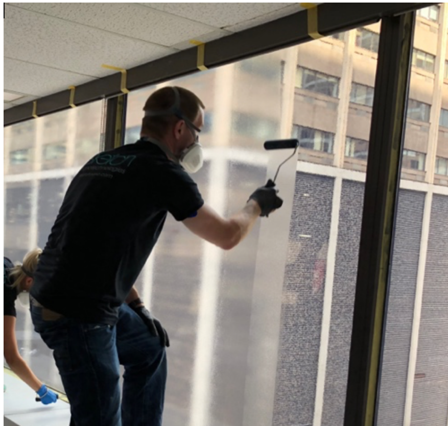
Figure 3.2: SNG-SC coating application on the glazing surface.
