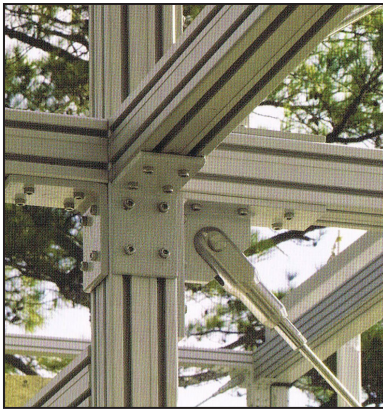
Fig 3.7.5 Aluminum frame with bolted connections
