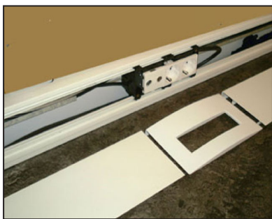
Fig 3.4.6 Open wall access panel with outlet cover and finish strip
