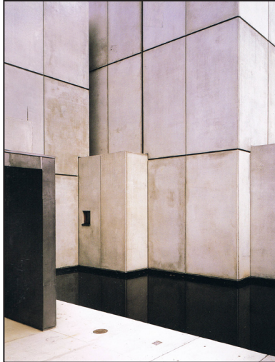
Fig 2.4.12 Peter Marino and Assoc., Datascape Corporation displays the intentional panelization of a surface through shadows of joints
