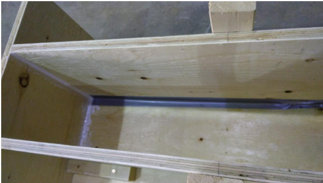
Figure 20: Formwork interior covered with a sealant (silicone) and duct tape
