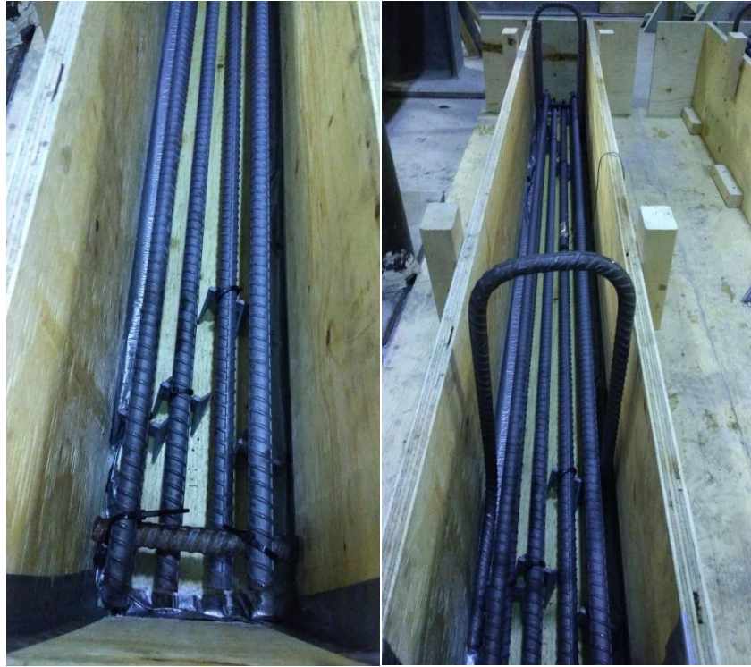
Figure 19: Reinforcement placement showing steel spacers and steel hooks
