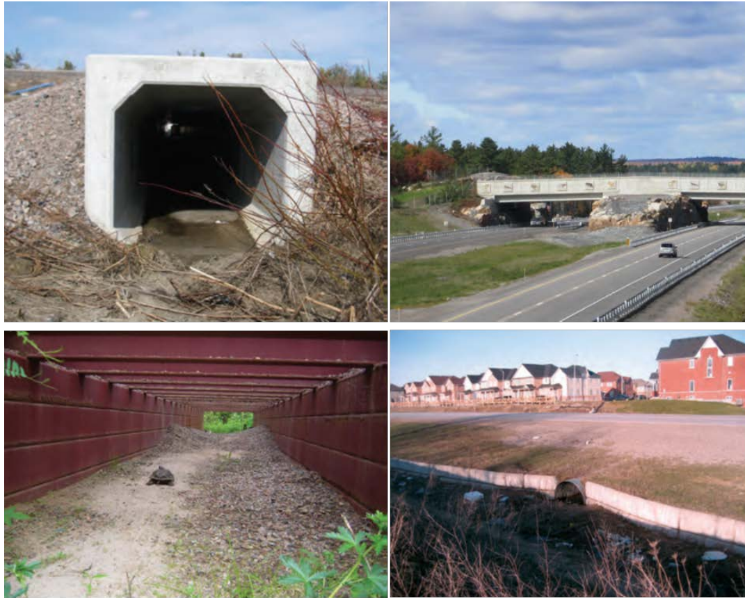
Figure 9: Images of examples of wildlife crossing structures in Ontario (top-left to bottom-right): box culvert underpass (©K. Gunson), 30m overpass on Hwy. 69 (©K. Gunson), open-grate tunnel (©A. Mui), concrete exclusion wall and culvert (©K. Gunson) (source: OREG, 2010)
